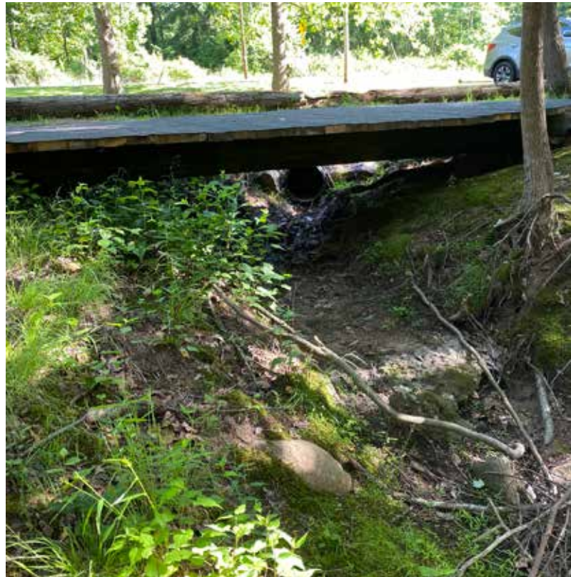
Currently, stormwater from Clarks Valley Road flows directly into Clarks Creek.
