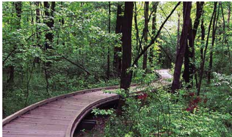
A recycled plastic timber boardwalk in a woodland wetland area.
