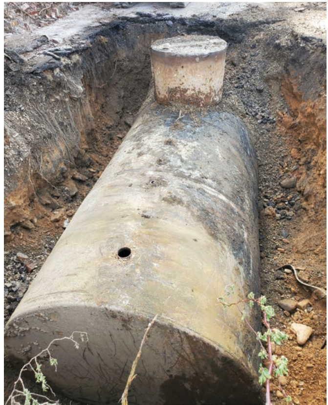
Excavating the UST
