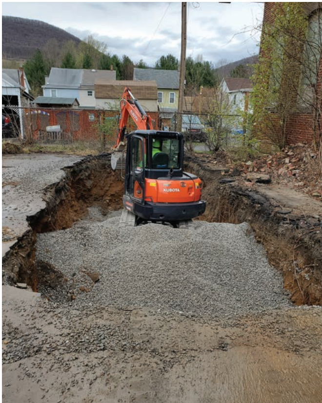
Clean 2B stone for backfill
