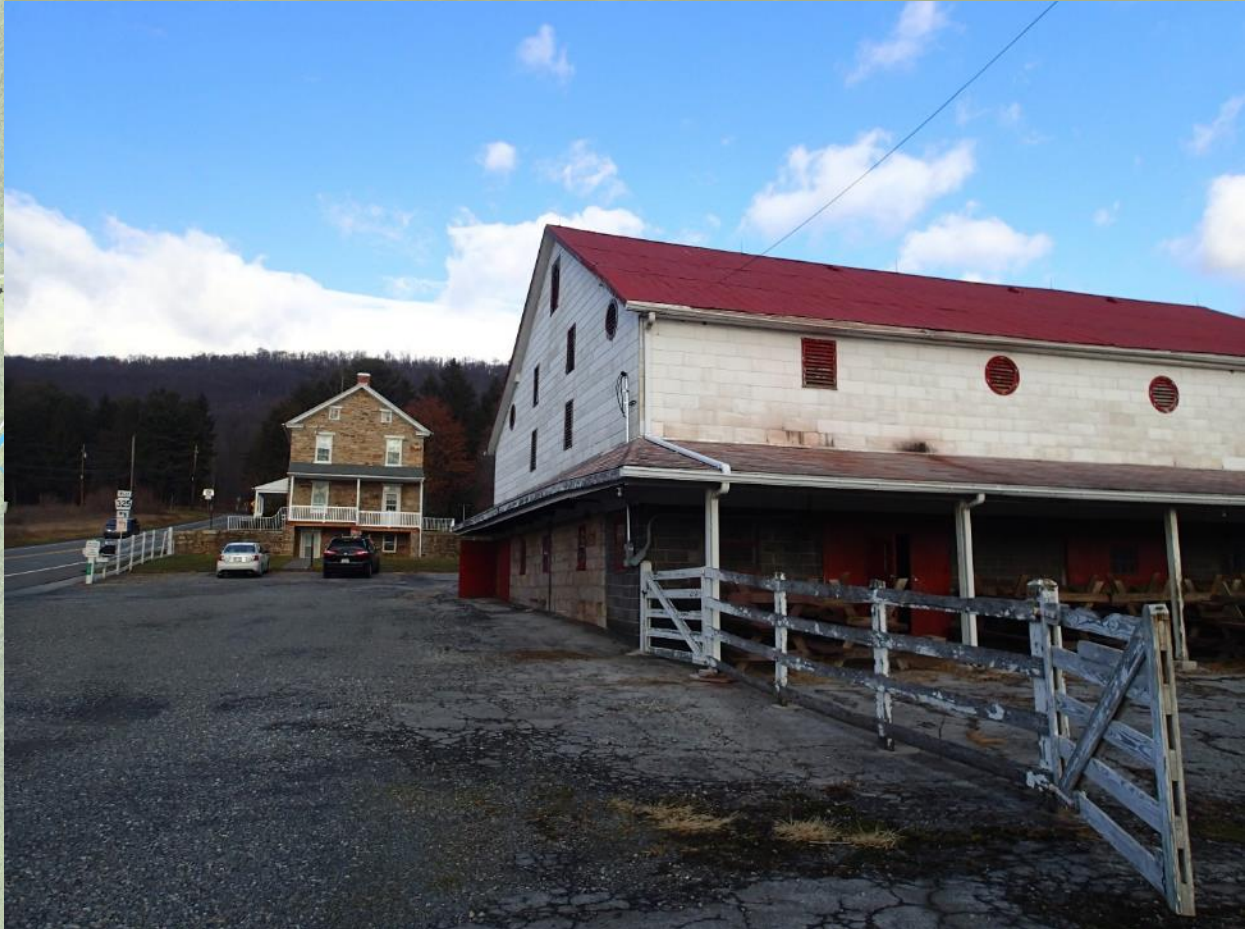
— — 1861 Peter's Mountain House and Barn along Peters Mountain Road
