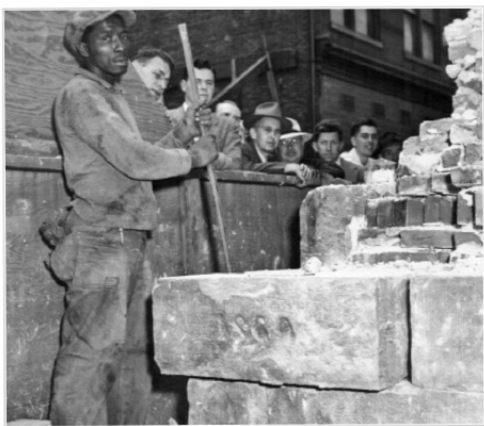
Dauphin County Courthouse Cornerstone Removal
